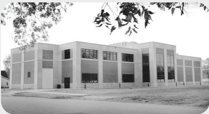
Construction Technology Facility at Vincennes University
