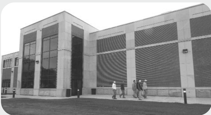
Construction Technology Facility at Vincennes University
